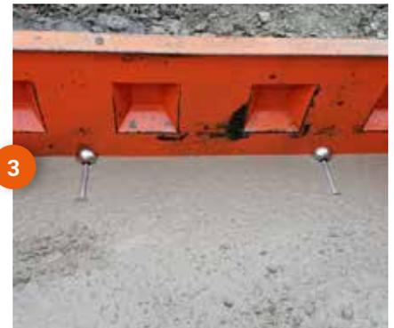
3 The anchor is cast in its entirety, be careful when vibrating the concrete
