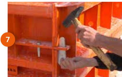
7 Removing pins and wedges
