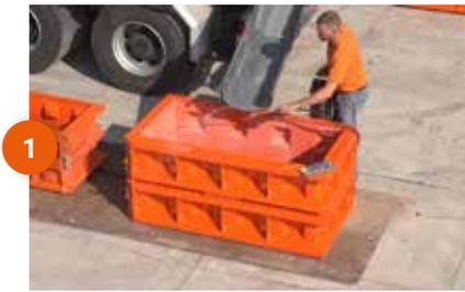
1 Place the mould on a leveled surface
